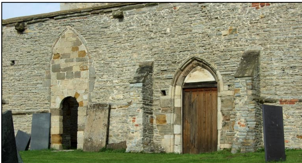
Figure 14. Part of the South Aisle with original porch door.
