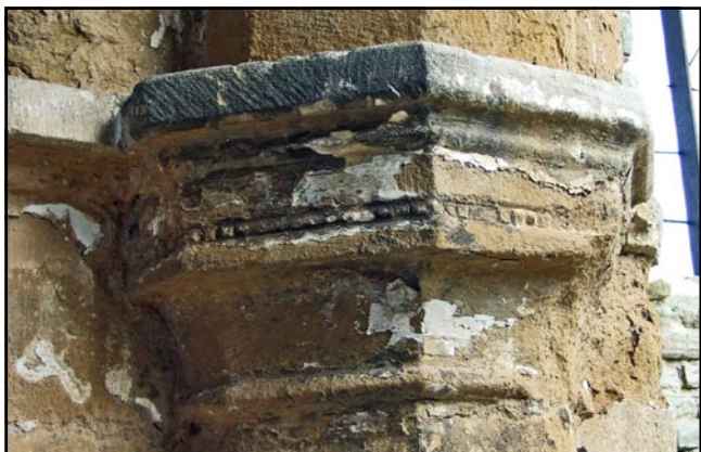
Figure 10. Nailhead decoration on the capitals of a column supporting the Tower's arches, with traces of old whitewash.
