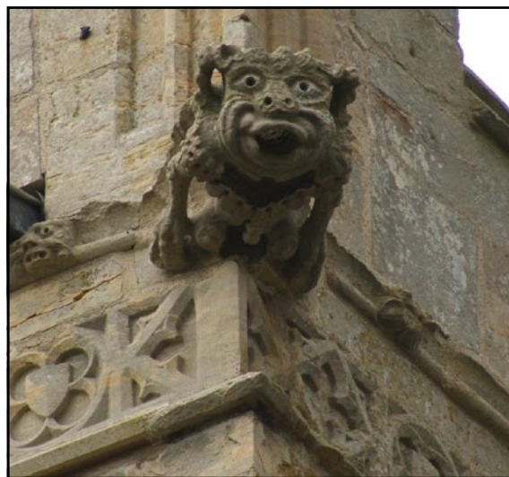
Figure 13. Gargoyle at SW corner of Tower, set above a carved frieze, both in Lincolnshire Limestone.
