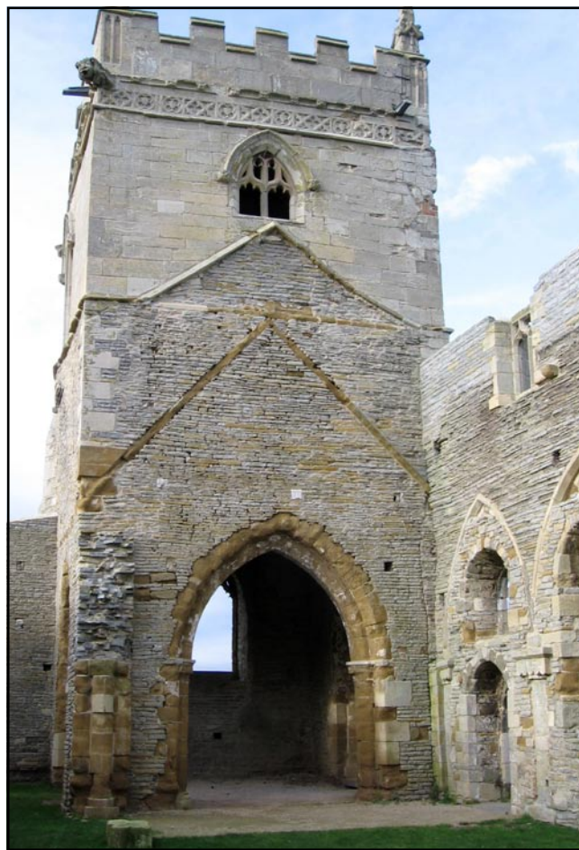
Figure 9. East Face of Tower with five faceted arch built of Sandrock (Early English style, C 13). The two ribs relate to original roof lines. The lower Sandrock rib ends just above the North Aisle Arches. The higher hipped rib consists of Lincolnshire Limestone and marks the building of the Clerestory and reconstruction of the Tower in the Perpendicular style (C 14).
