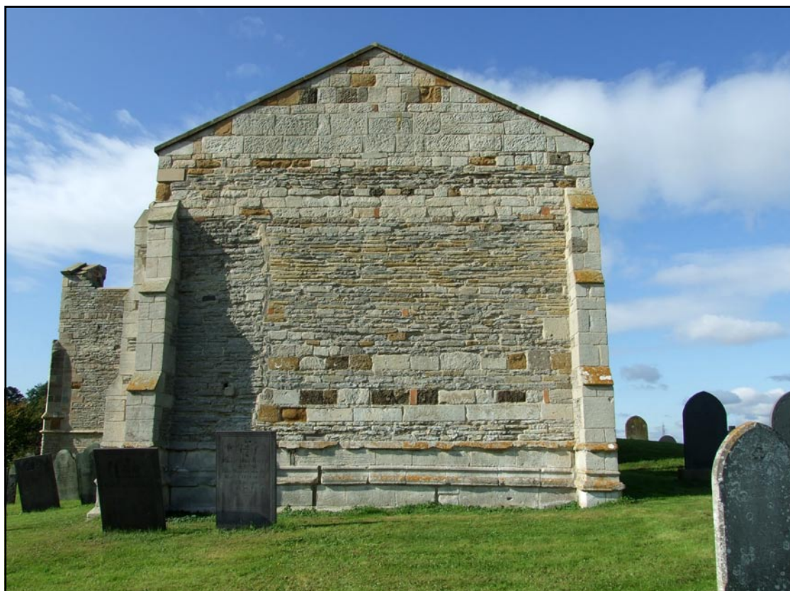
Figure 17. The east wall, rebuilt without a window.
