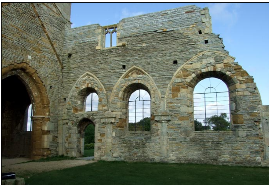
Figure 7. North Arcade Nave Wall. The two and a half rounded columns with scalloped capitals, all Lincolnshire Limestone, are typically Norman. Subsequently the North Isle was raised with the insertion of ribbed pointed arches mostly oolite with some sandstone. The first two are set below the ironstone roof rib of the tower, but the third is taller and wider. Georgian style windows were inserted when the arcade became the Nave Wall.
