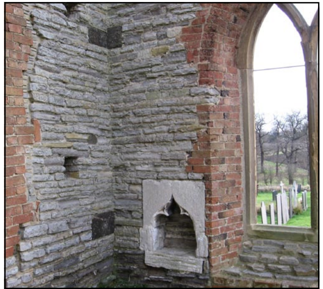
Figure 3. Southeast corner of the Chancel with Blue Lias rubblestone enclosing a piscina carved from a block of oolite adjacent to a C19th window.
